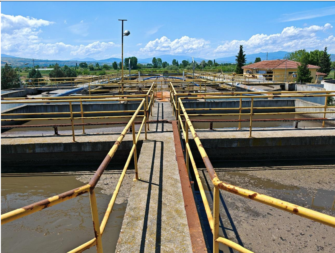
Erbaa WWTP of Anaerobic and Aeration Tanks
